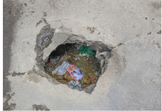
Figure 4: A pit in peri-urban Lusaka with solid waste visible. The pit has sat filled and the toilet unused for several months.
